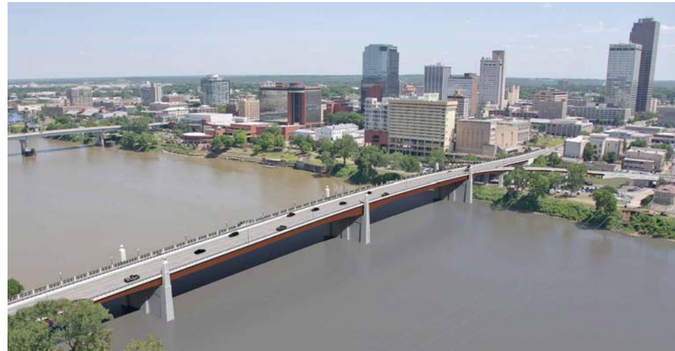
Alternative 3A – Plate girder on offset alignment-retain existing bridge
